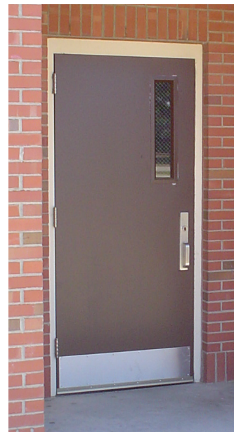
Ft Bragg Barracks Stairwell Door
